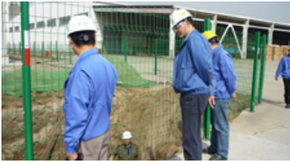
Site Tour Inspection
