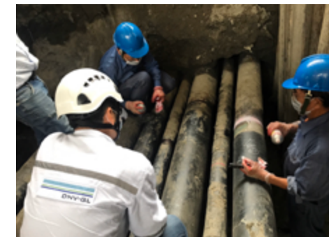
Excavation verification and inspection of pipelines
