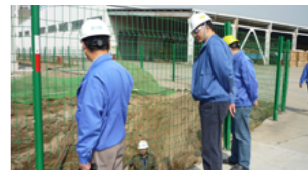
Site Tour Inspection
