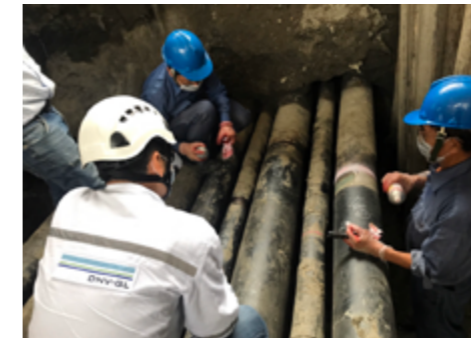
Excavation verification and inspection of pipelines
