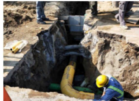
Excavation verification and inspection of pipelines
