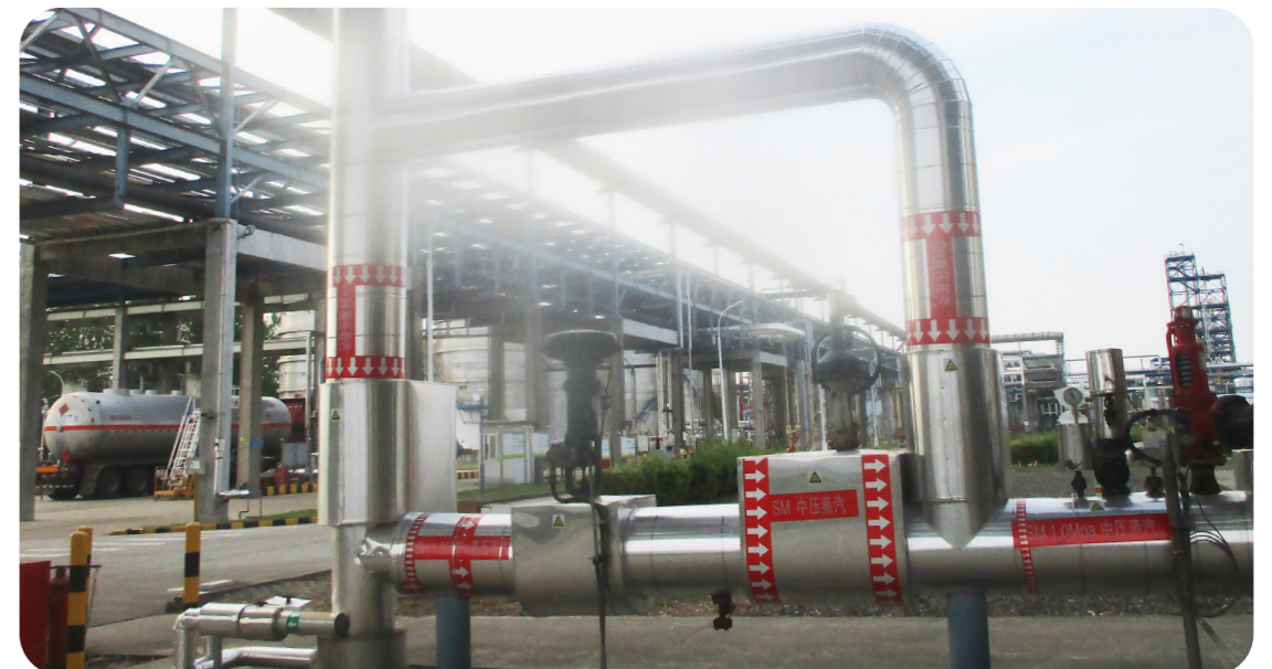
Nantong Industrial and TSRC-UBE SEBSSIS Steam pipes replacement
