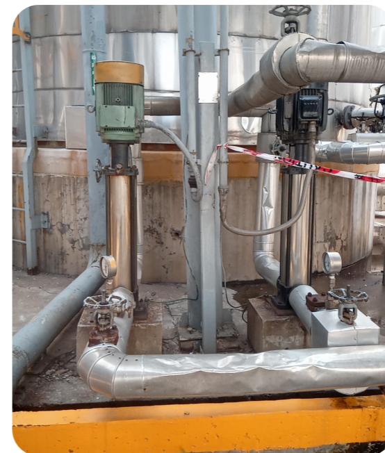
Nantong Industrial and TSRC-UBE SEBSSIS Steam pipes replacement
